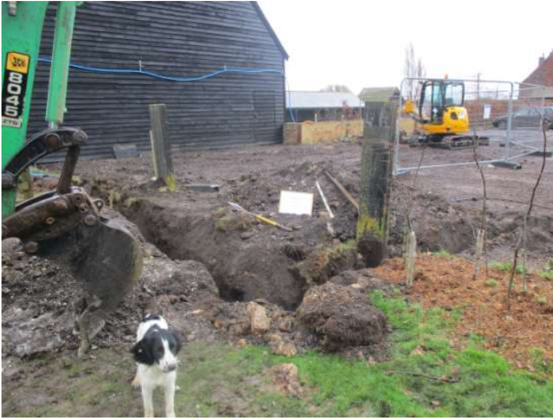
Plate 4. Excavation starting on the remainder of the foundation trenches
