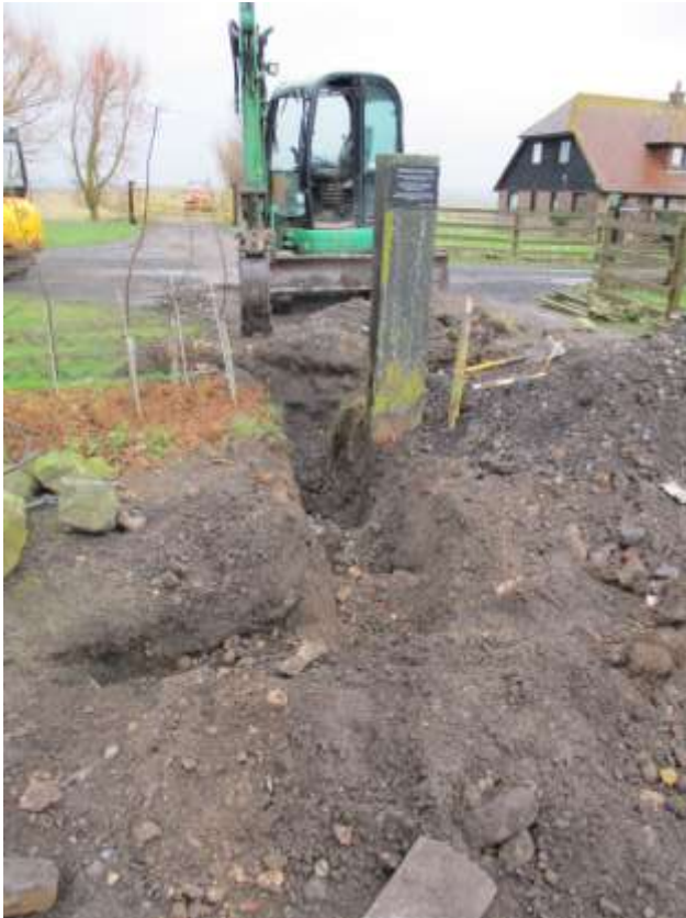
Plate 5. Cutting through made up ground
