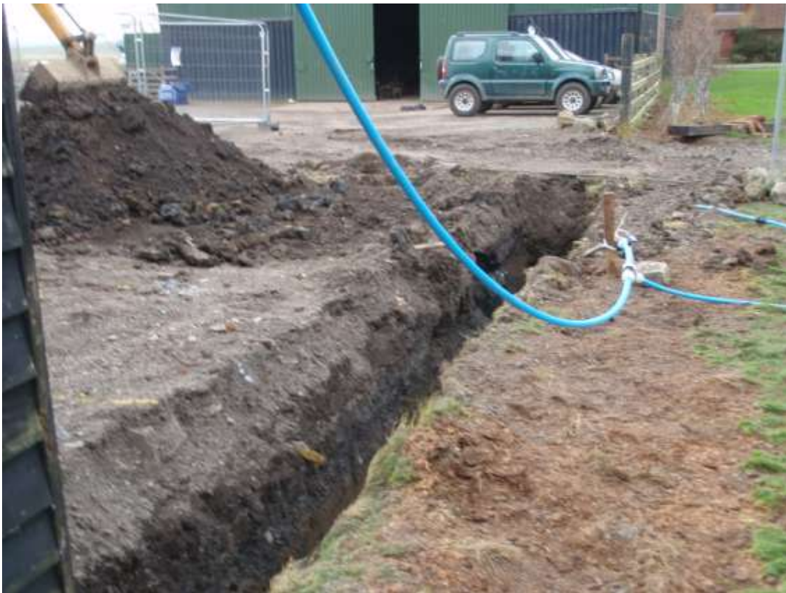
Plate 3. Foundation trench on the north side- note repaired water pipe
