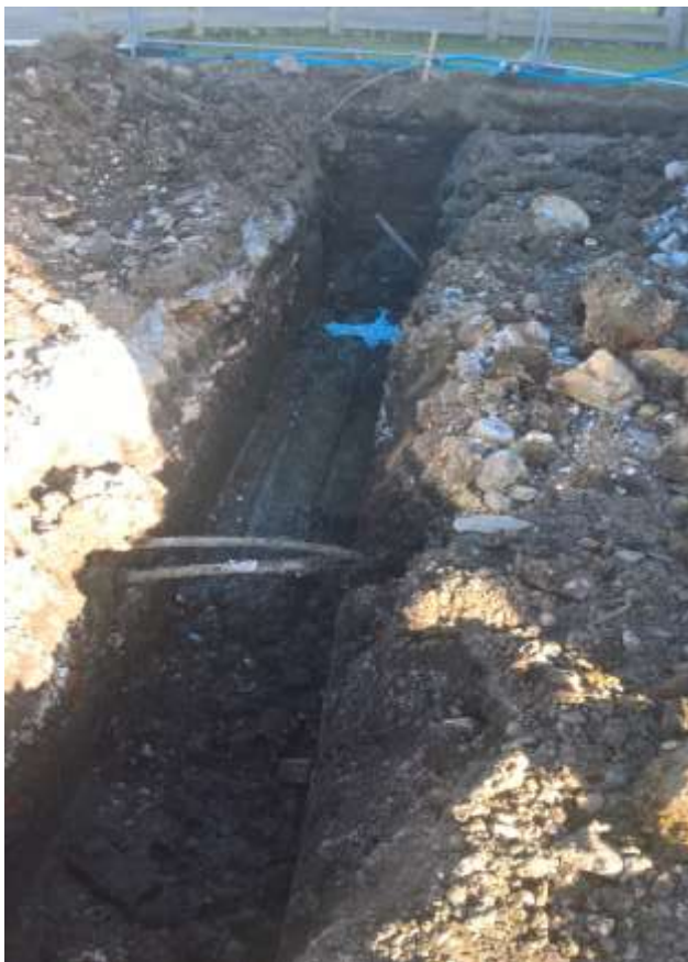
Plate 7. Completed foundation trenches
