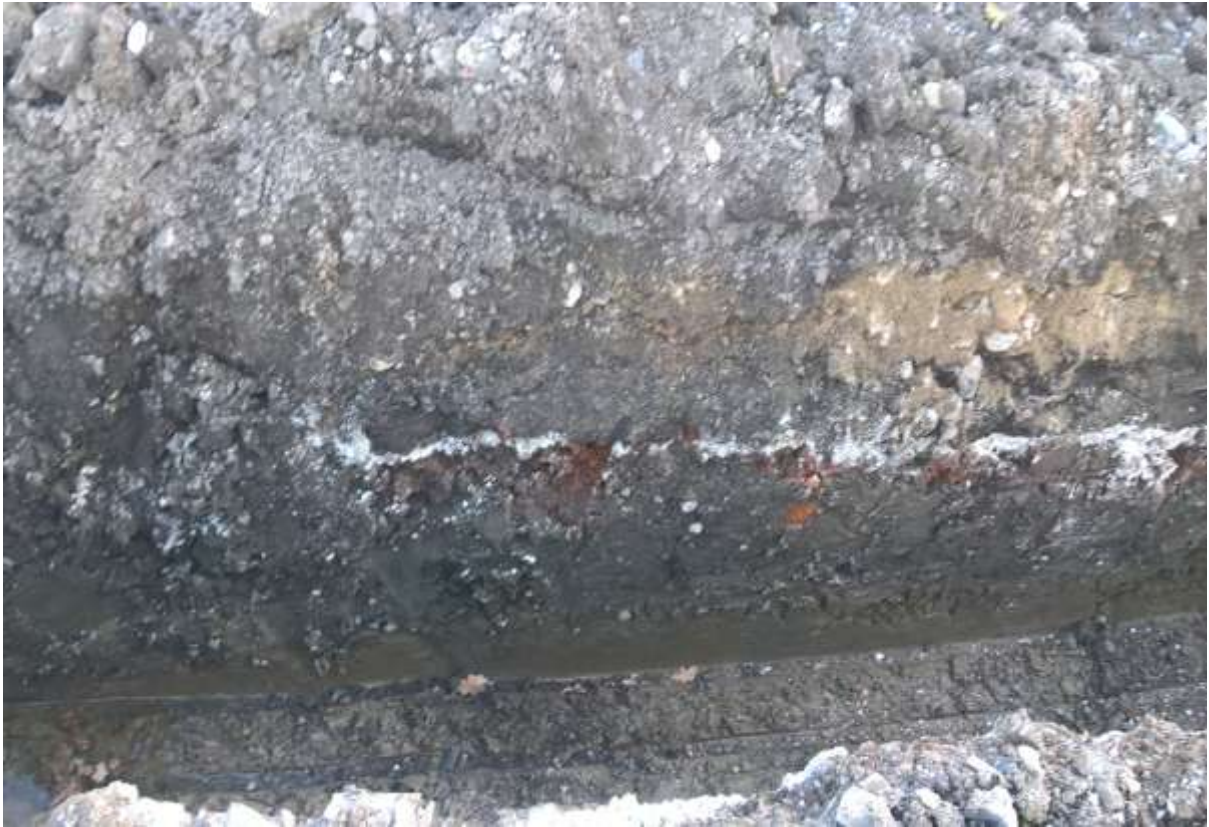
Plate 6. Completed foundation trenches
