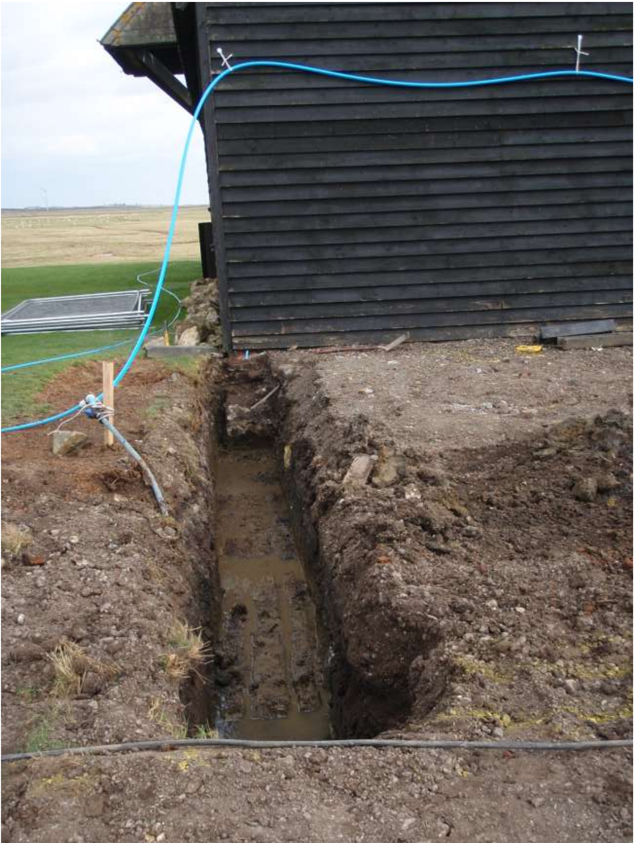
Plate 3. Completed foundation trench on the north side
